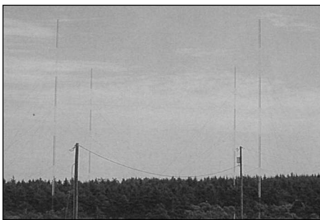
Antény VY2ZMM - 4 square pro 160m (op. K1ZM, K2WI, WW2Y)
